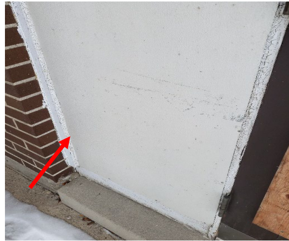
Photograph No. 30 Non-Asbestos white caulking (Sample Group 25017022-ASB-28A-C). Exterior doors & windows.
