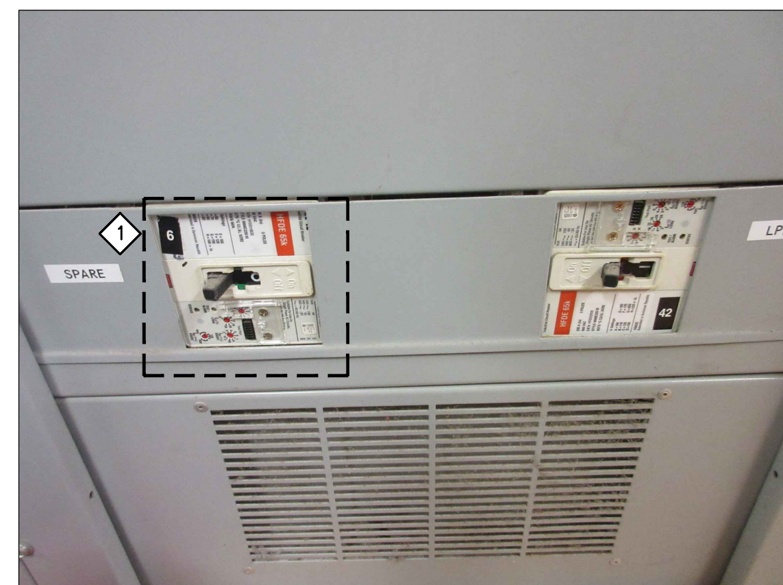
SPARE CIRCUIT BREAKER 06 NTS
