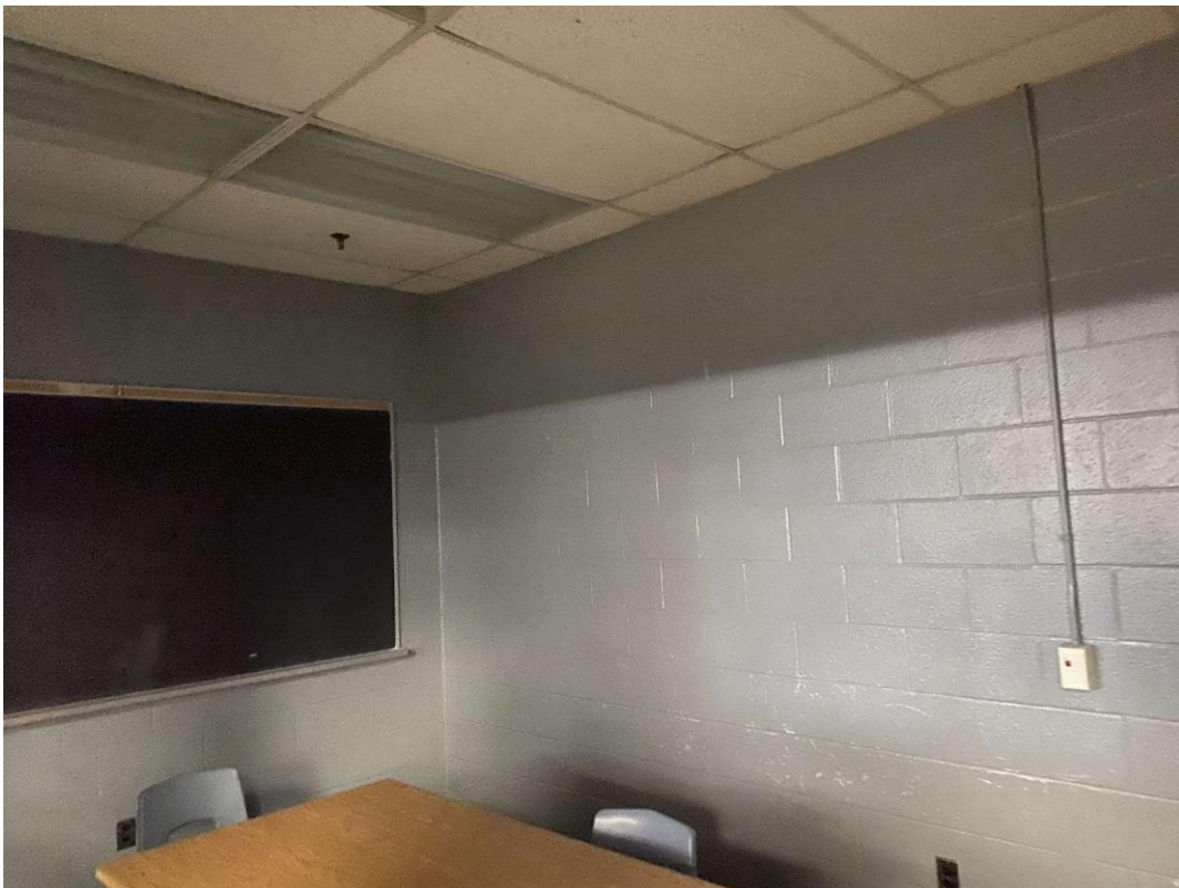
L0003(Lead, None), White and blue concrete block, Wall, Learning Commons / Atrium / Foyer / Study Rooms (Location #: 4)
