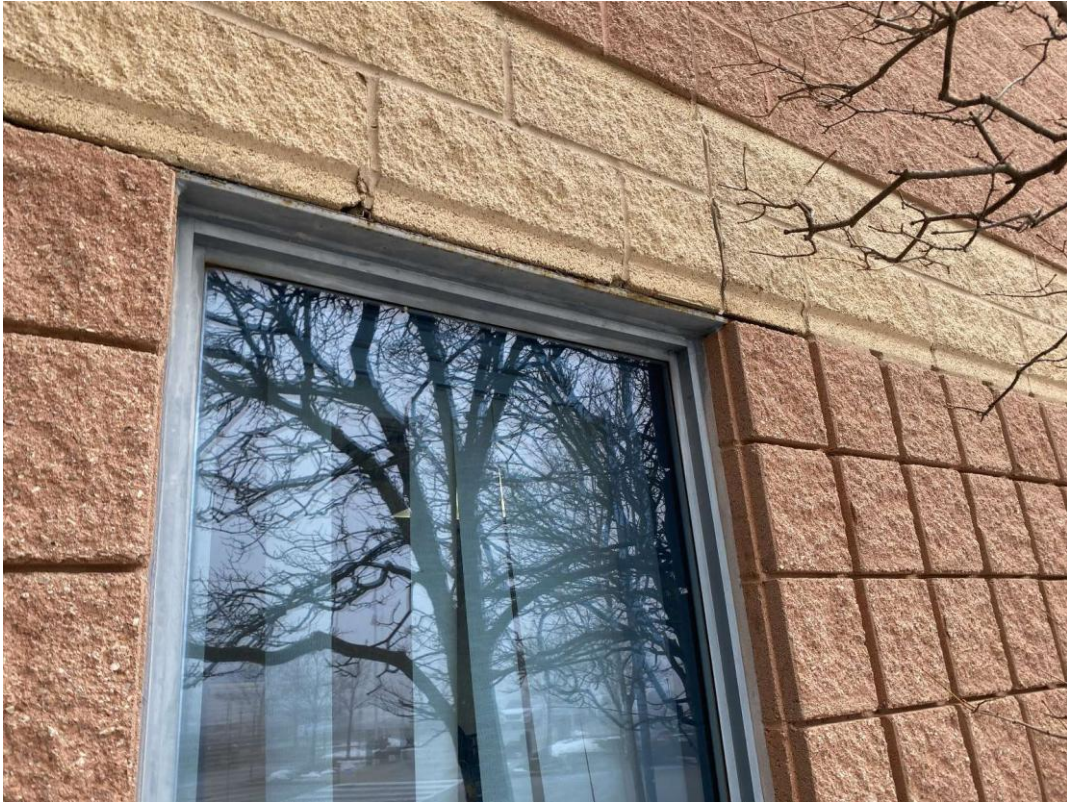
S0010A (None), White, Other, Window, Caulking, Exterior 1997 (Location #: 18)
