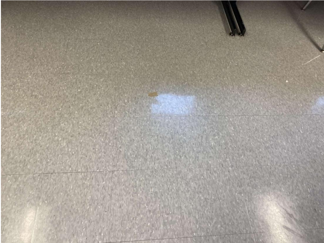
S0006A (None), 12x12 grey with white and dark grey fleck, Floor, Vinyl Floor Tile and Mastic, Play Rooms / Co-op Education (Location #: 6)
