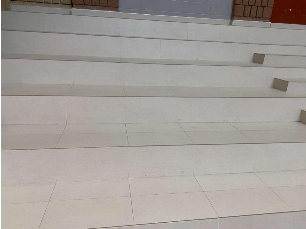
S0001A (None), 12x24 white and grey, Floor, Thin-set, Learning Commons / Atrium / Foyer / Study Rooms (Location #: 4)
