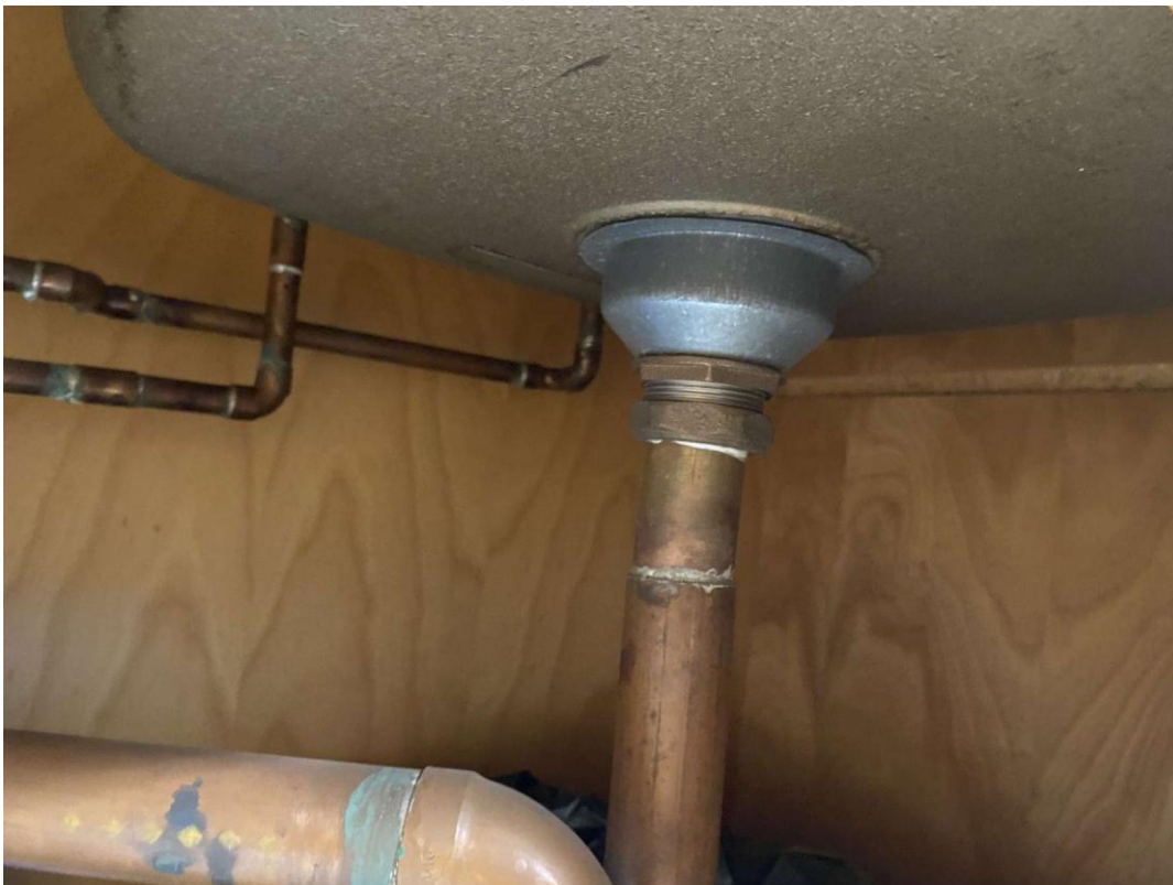
S0009A (Confirmed Asbestos), Other, Sink, Mastic, Gold, Science Labs and Classrooms (Location #: 12) Greenhouse
