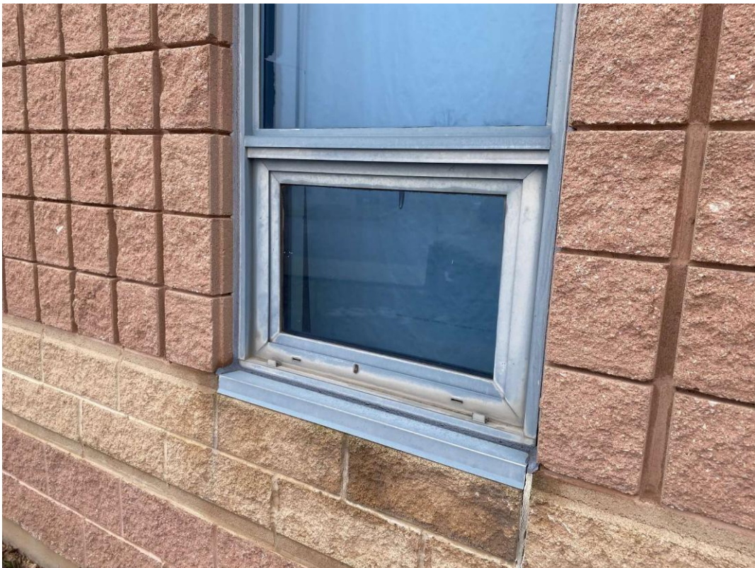
S0011A (None), White, Other, Window, Caulking, Exterior 1991 (Location #: 19)
