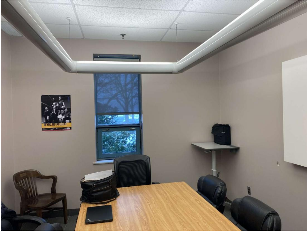
L0005(Lead, None), Brown, Wall, Offices (Location #: 3)
