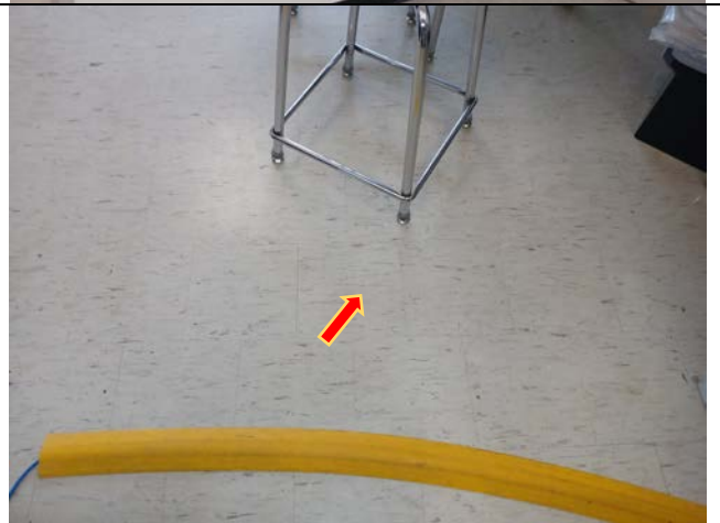
Photograph 2. View of the previously identified asbestos-containing VFTs, 9"x9", beige with brown streaks and associated black mastic on the floor in Work Room 203 on the 2 nd floor at the Subject Location.
