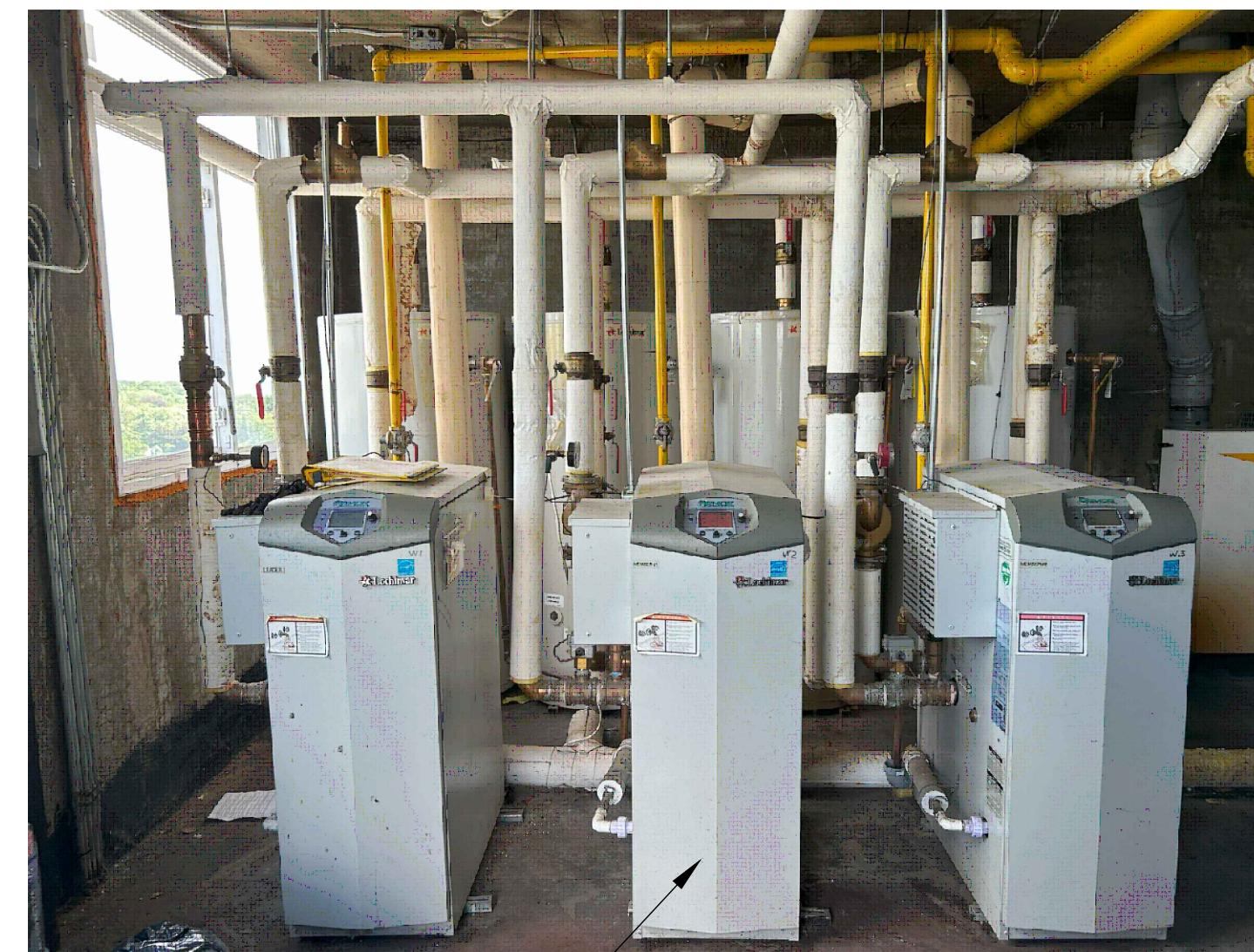
DEMOLISH & REMOVE ALL EXISTING DOMESTIC HOT WATER BOILERS (TYP. OF 3)
