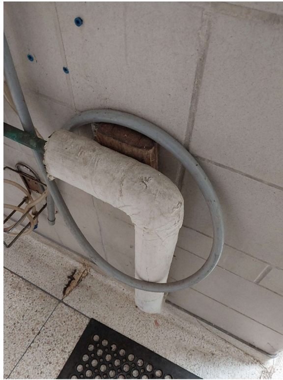
Photograph No. 3 – Parging was observed on two fittings within Room 1044A. The parging was sampled (S08A,B,C) and is asbestos-containing. Additional fittings may also be present in concealed spaces. Pipe straight insulation was observed to be fiberglass and is non-asbestos.
