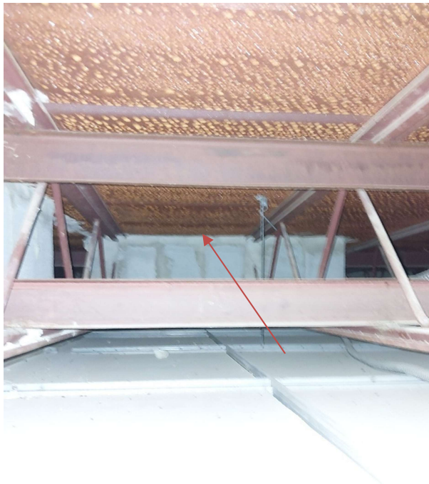
Photograph No. 3 – Parging was observed on two fittings within Room 1044A. The parging was sampled (S08A,B,C) and is asbestos-containing. Additional fittings may also be present in concealed spaces. Pipe straight insulation was observed to be fiberglass and is non-asbestos.
