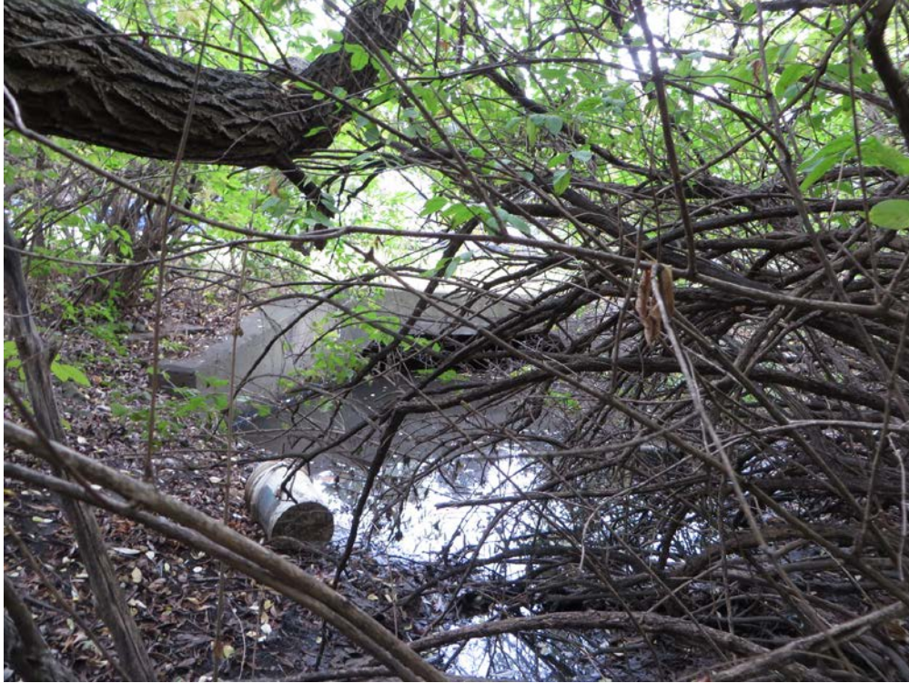
Photo 5: Viewing south towards Barton street at Watercourse 4 storm sewer inlet.
