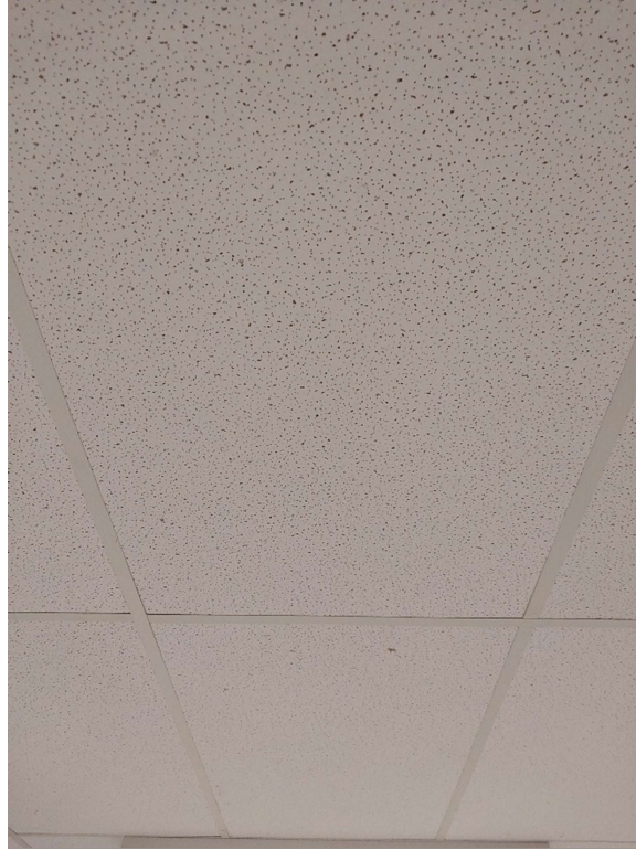
Photograph No. 3 – 2'x4' small fissure random pinhole ceiling tile was observed throughout the building. The ceiling has a post-1990 date stamp is not considered asbestos-containing.
