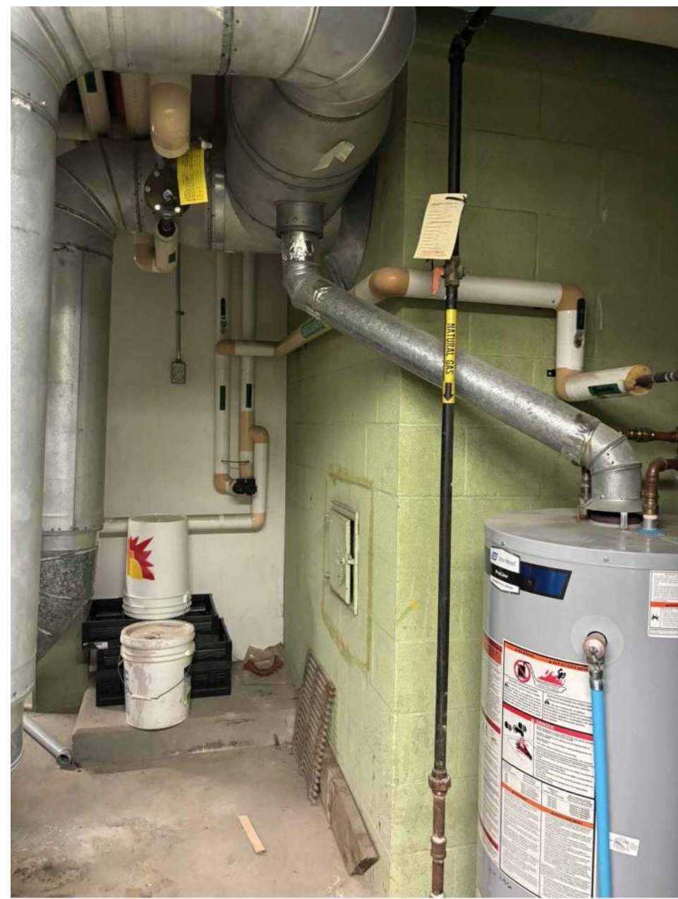
REFERENCE IMAGE - EXISTING CHIMNEY
