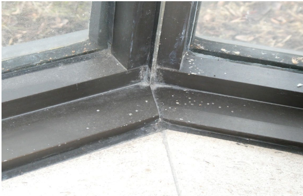
PHOTO #18 – WINDOW SILL DETAIL @ W1A / W1B CORNER
