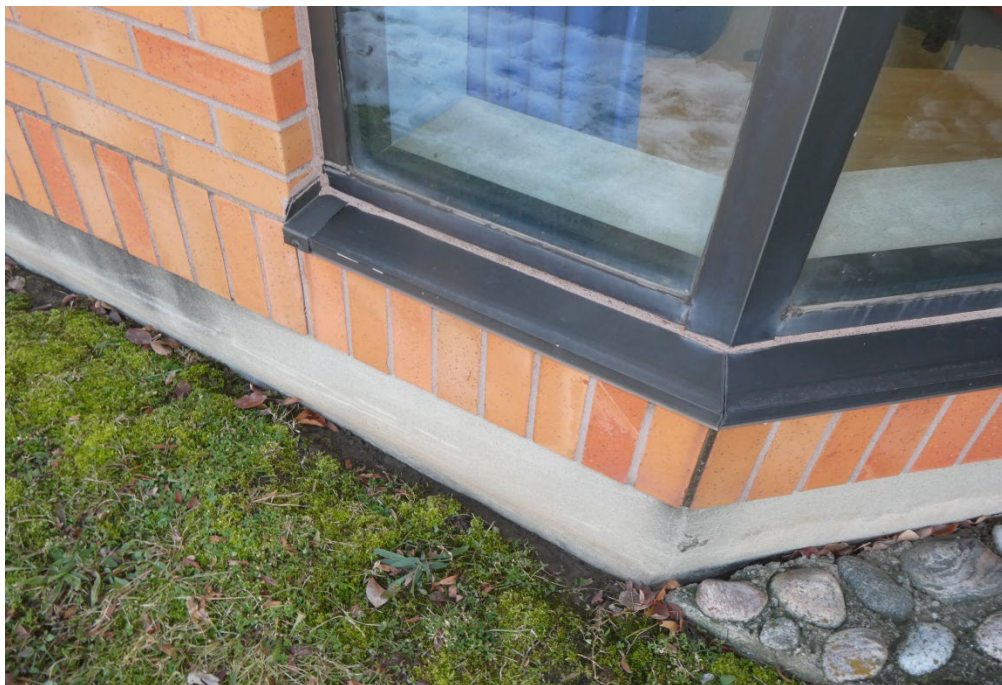
PHOTO #12 – EXTERIOR SILL DETAIL @ W1A WINDOW
