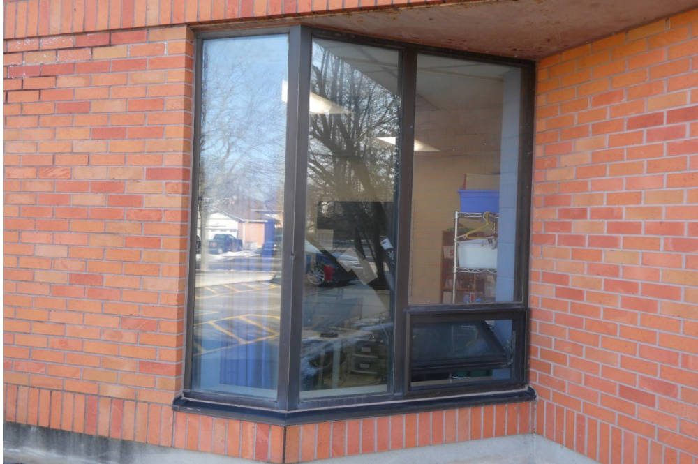
PHOTO #9 – TYPICAL VIEW OF W1A WINDOW
