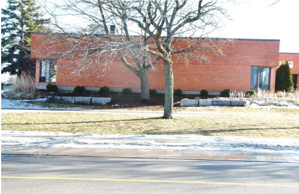
PHOTO #1 – VIEW OF PARTIAL NORTH (FRONT) ELEVATION
