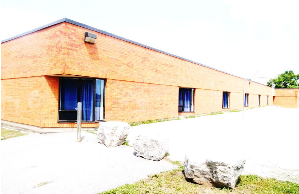
PHOTO #5 – VIEW OF PARTIAL SOUTH (REAR) ELEVATION
