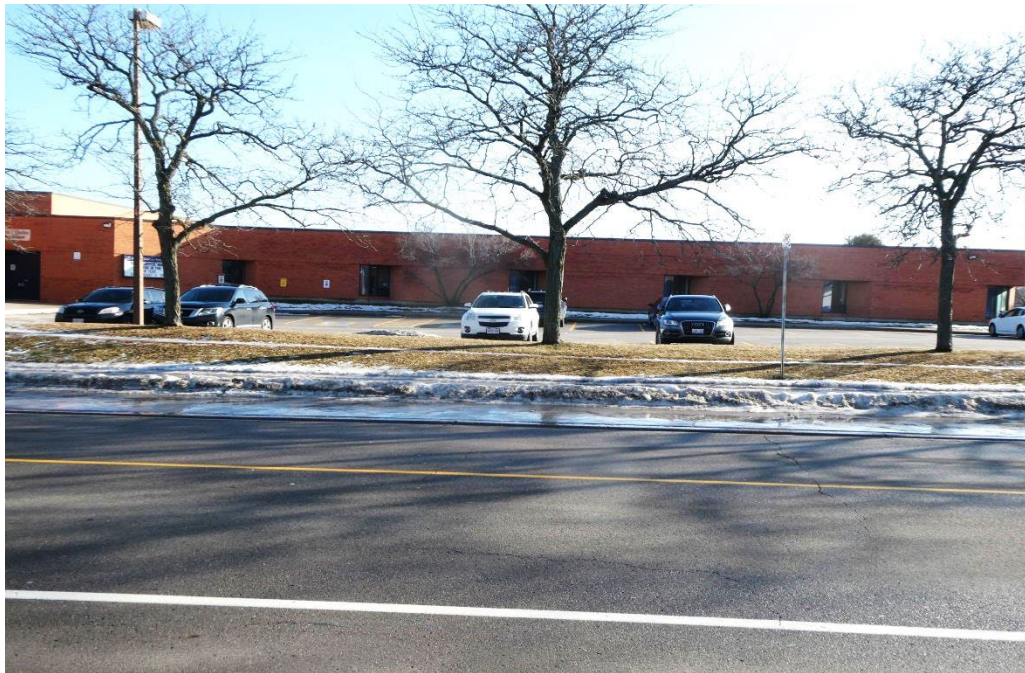
PHOTO #2 – VIEW OF PARTIAL NORTH (FRONT) ELEVATION
