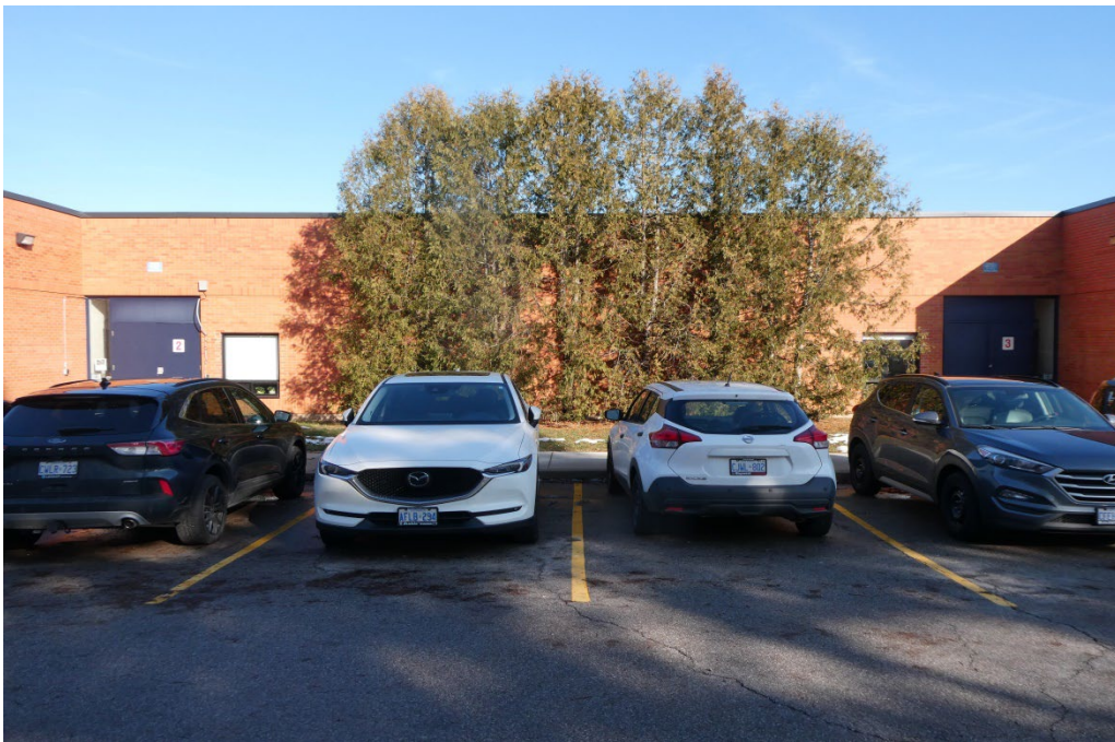
PHOTO #4 – VIEW OF PARTIAL WEST ELEVATION
