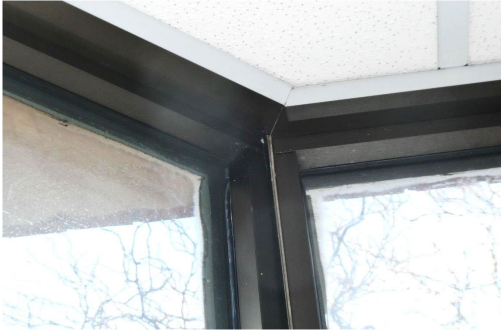
PHOTO #17 – WINDOW HEAD DETAIL @ W1A / W1B CORNER
