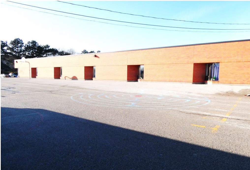
PHOTO #6 – (ALT) VIEW OF PARTIAL SOUTH (REAR) ELEVATION
