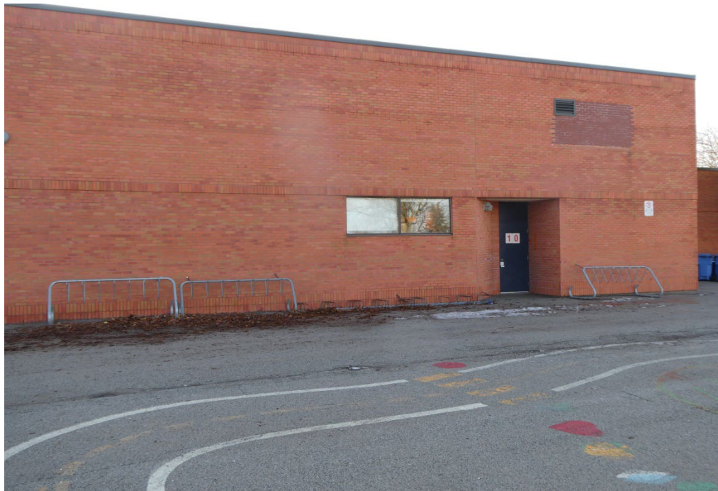
PHOTO #8 – VIEW OF PARTIAL EAST ELEVATION
