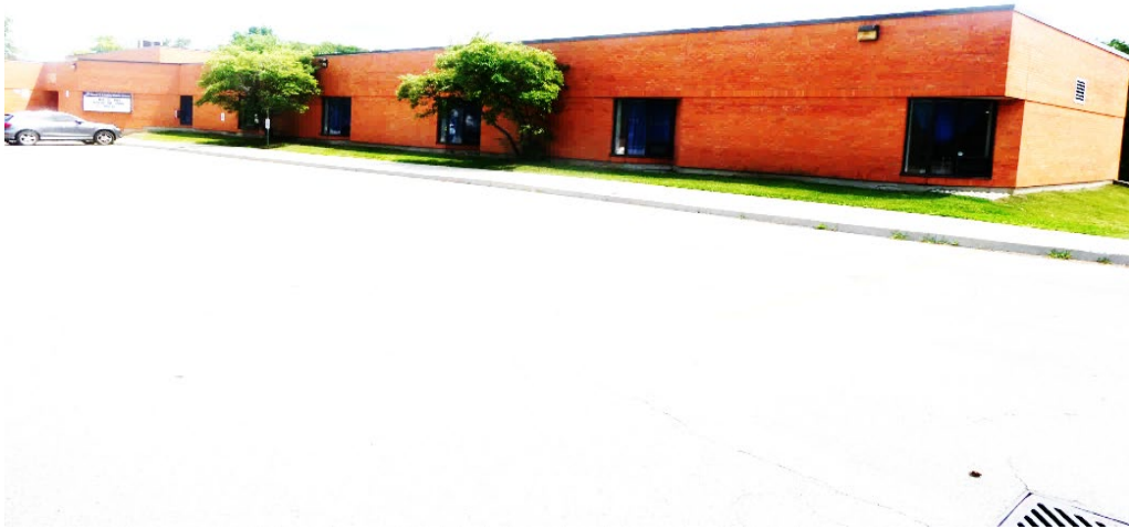
PHOTO #3 – (ALT) VIEW OF PARTIAL NORTH (FRONT) ELEVATION
