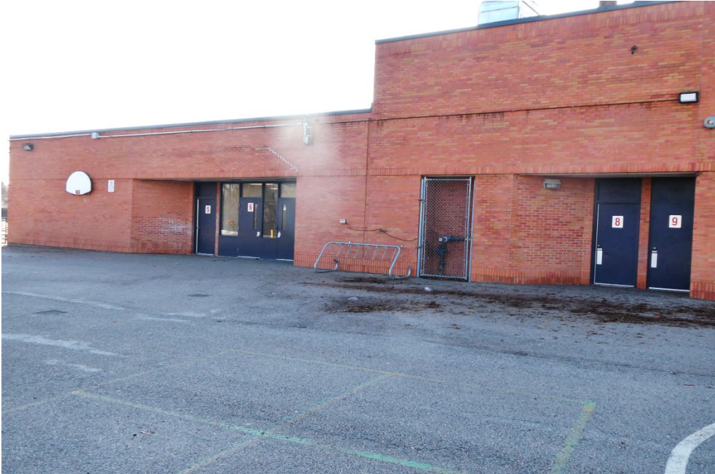
PHOTO #7 – VIEW OF PARTIAL EAST ELEVATION
