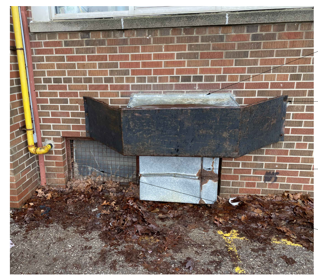
8 PHOTO - BASEMENT VENT REPLACEMENT A4.1
