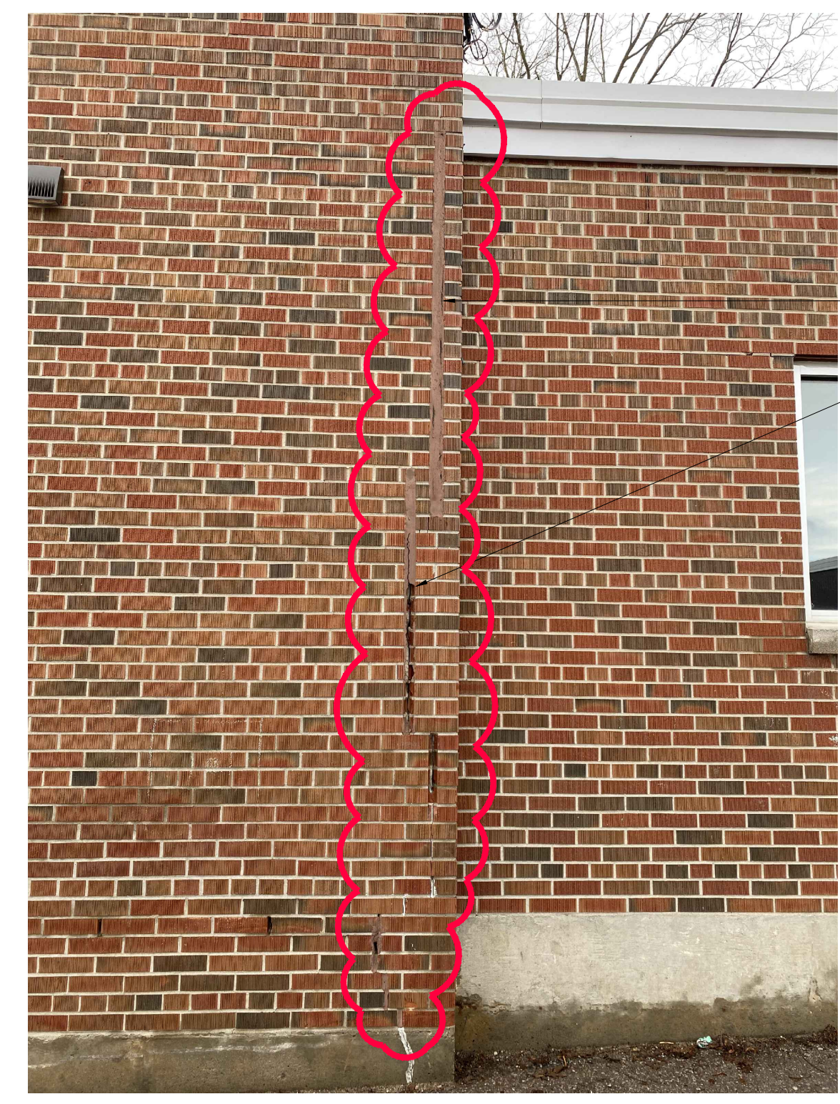
6 PHOTO - MASONRY REPAIRS A4.1
