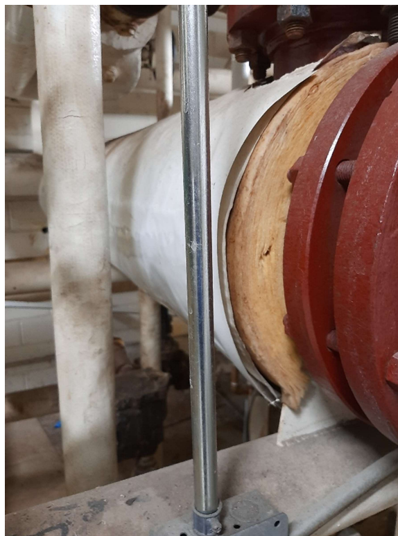
Photograph No. 8 – Pipe straights throughout the primary boiler room were observed to be comprised of fiberglass.
