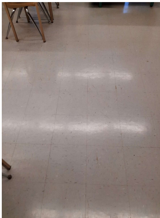
Photograph No. 14 – 12"x12" Vinyl Floor Tile was sampled from room 126 (S17A,B,C) and is not asbestos containing; however, the mastic is asbestos containing.
