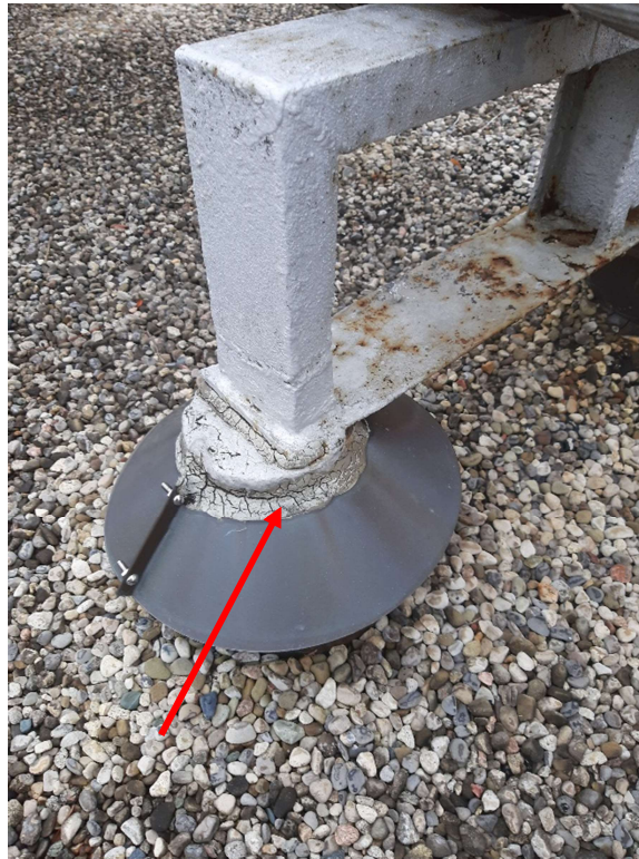
Photograph No. 3 – The sealant associated with the steam pipe mounting was sampled (S02A,B,C) and is not asbestos-containing.
