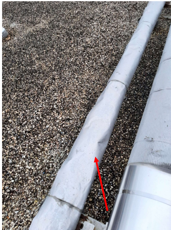
Photograph No. 2 – The insulation within the smaller steam pipe adjacent to the large steam pipe was inaccessible and therefore is suspected to contain asbestos.
