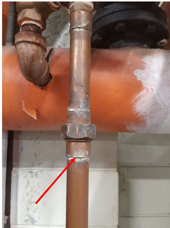
Photograph No. 6 – Suspect lead containing solder on copper pipe connections were observed within the secondary boiler room.
