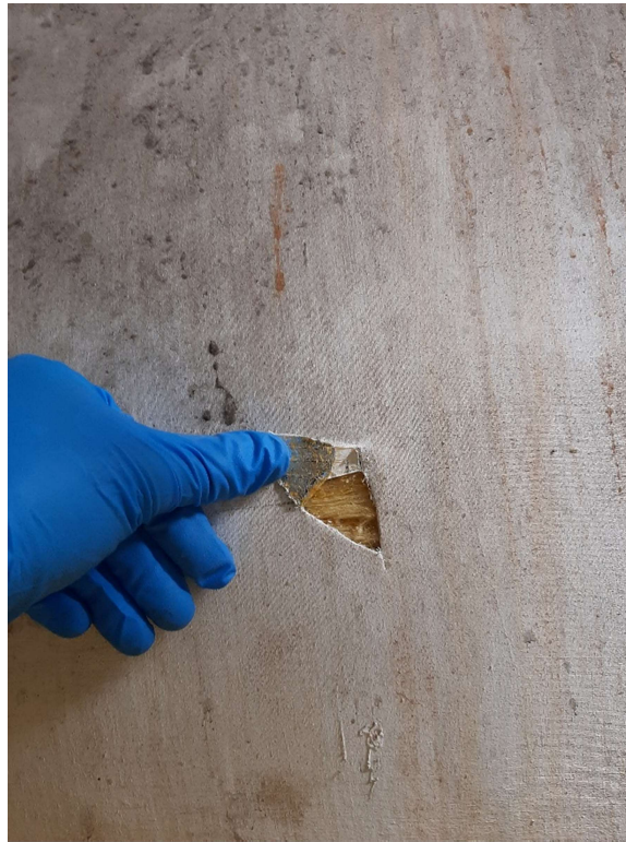
Photograph No. 9 – The insulation on the large white heat exchanger/storage tank was observed to be fiberglass.
