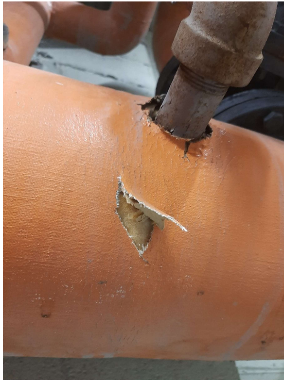
Photograph No. 5 – Pipe straights were inspected within the secondary boiler room and were comprised of fiberglass.
