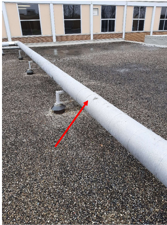
Photograph No. 1 – The insulation within the large steam pipe on roof section 102 was sampled (S01A,B,C) and is asbestos-containing.
