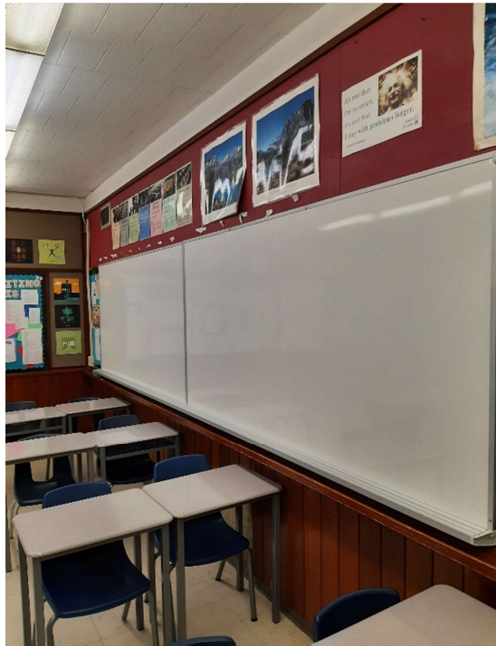
Photograph No. 22 - Suspect asbestos-containing mastics may be present underneath classroom whiteboards and tackboards.
