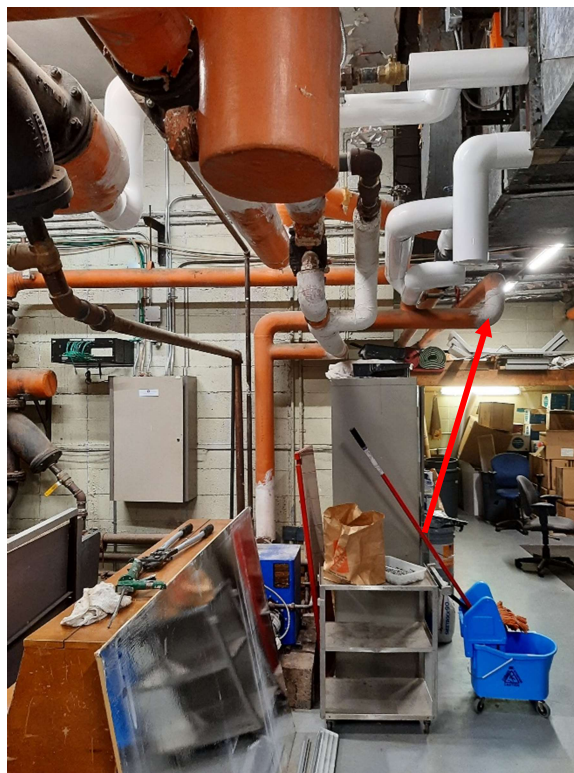
Photograph No. 4 – Pipe elbows within the secondary boiler room were sampled (S03A,B,C) and are asbestos-containing.
