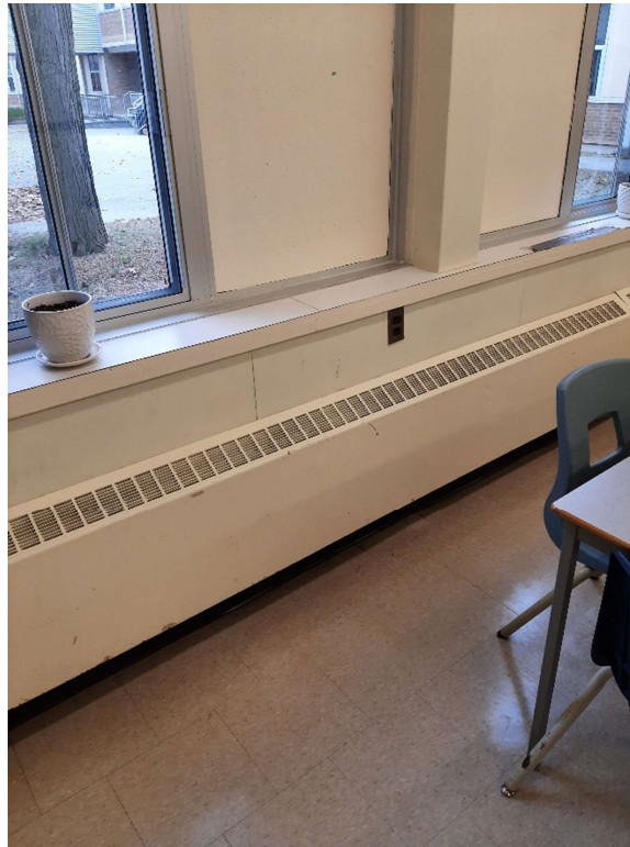
Photograph No. 20 - Interior sealant was sampled (S10A,B,C) and is not asbestos-containing. The cream paint on interior walls was sampled (LP04) and is low level lead-containing.
