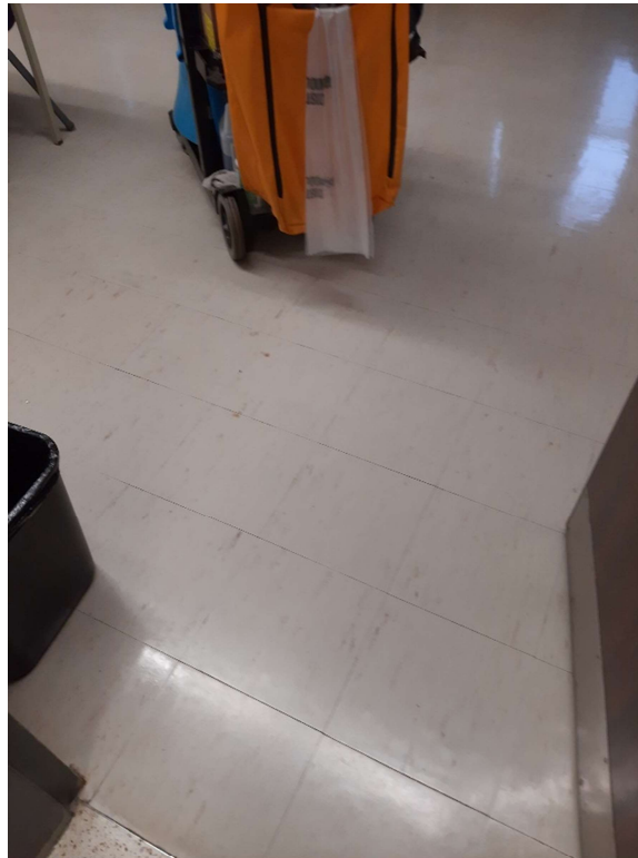
Photograph No. 13 – 12"x12" Vinyl Floor Tile was sampled from room 123 (S16A,B,C) and are not asbestos-containing; however, the associated mastic is asbestos-containing.
