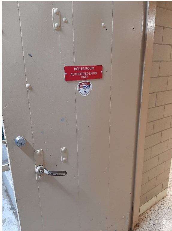
Photograph No. 11 – Fire doors were observed at the primary boiler room and are suspected to contain asbestos insulation.
