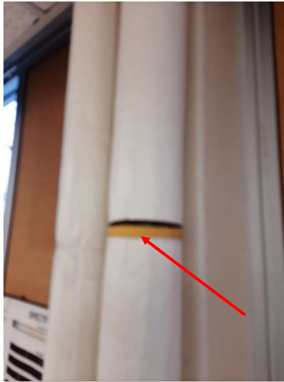
Photograph No. 24 - Fiberglass pipe straights were observed in classrooms throughout the interior.
