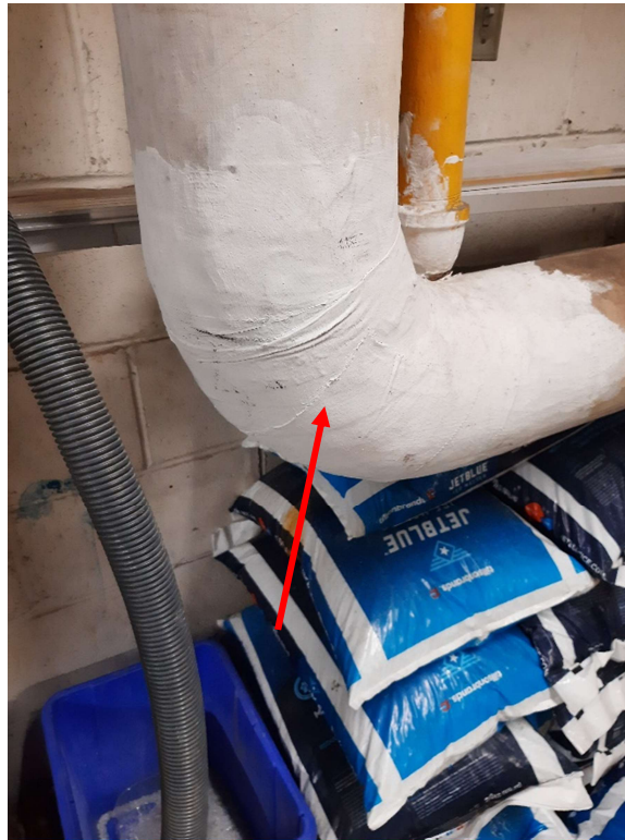
Photograph No. 7 – Pipe elbows within the primary boiler room were sampled (S06A,B,C) and are asbestos-containing.
