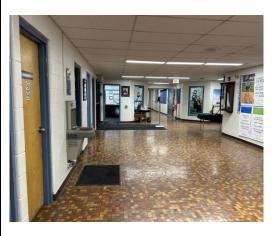
**Figure 1:** Examples of different ACM ceramic tile mortar base to be removed.
