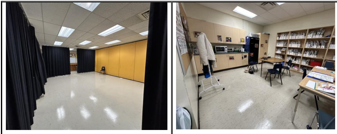
Figure 1: Examples of different ACM vinyl floor tile systems to be removed.
