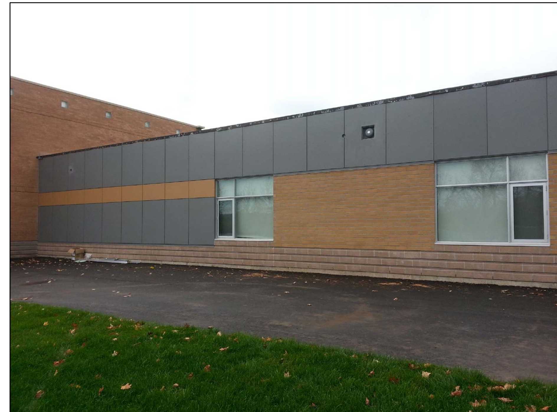
BUILDING ELEVATION - DURING CONSTRUCTION FROM 2013
