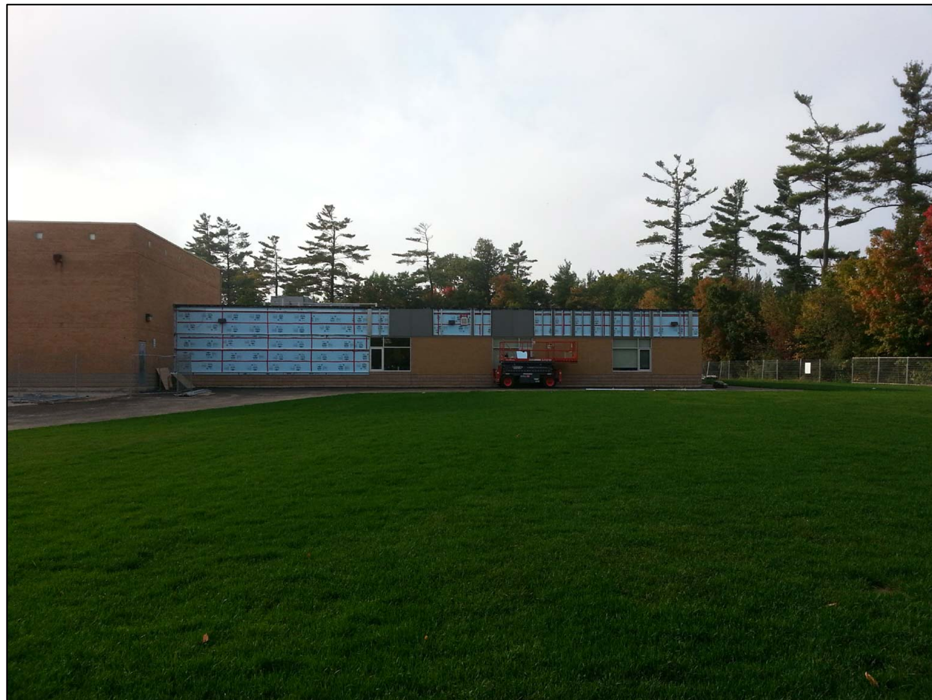
BUILDING ELEVATION - DURING CONSTRUCTION FROM 2013
