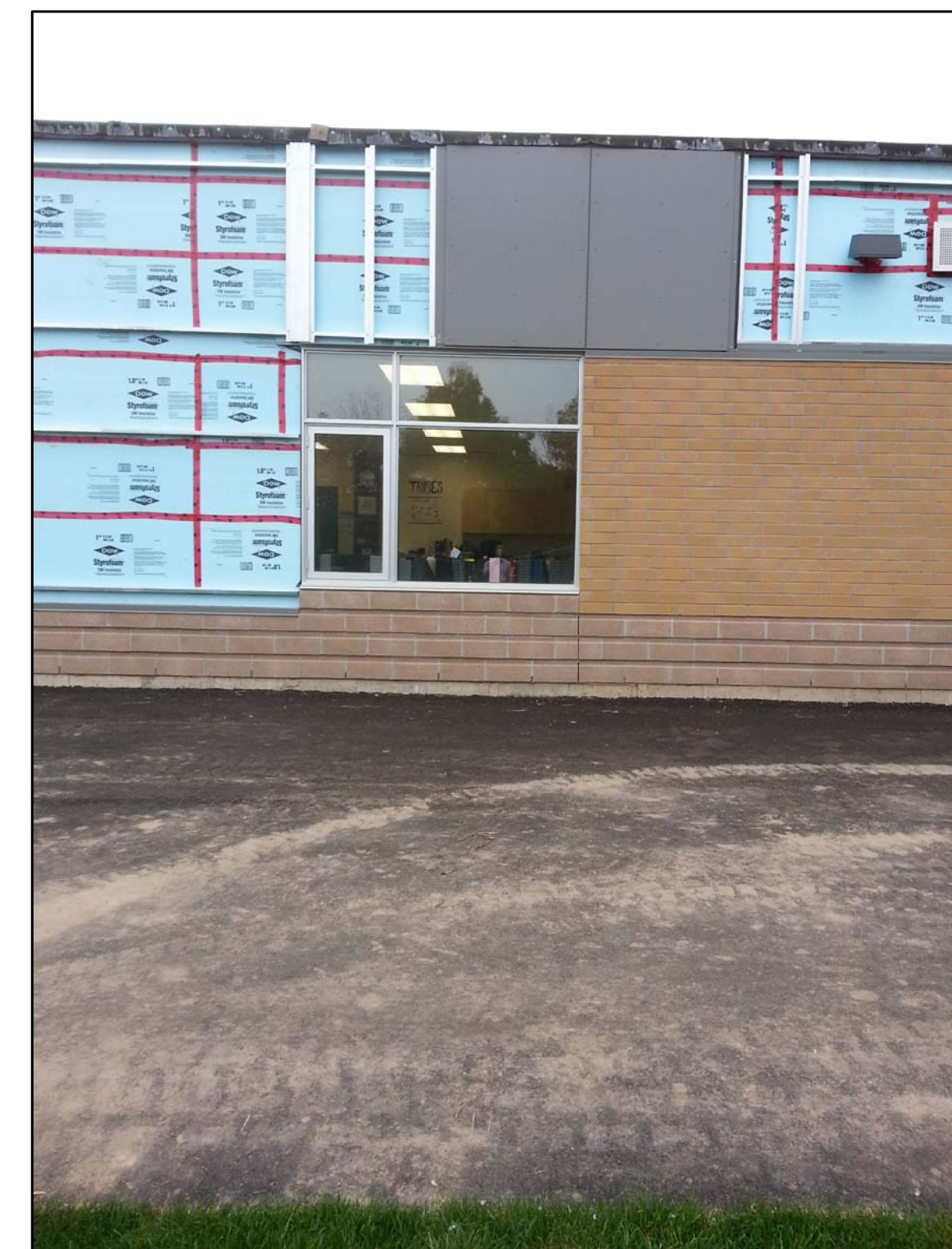
BUILDING ELEVATION - DURING CONSTRUCTION FROM 2013
