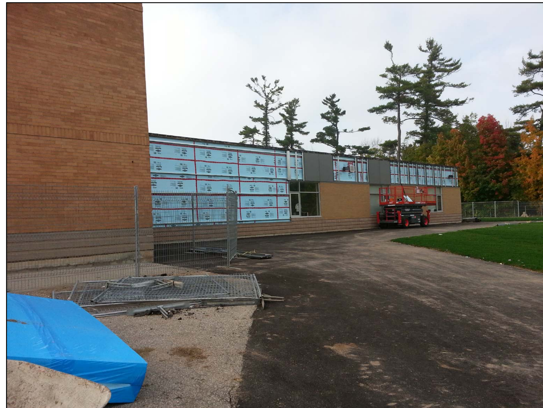
BUILDING ELEVATION - DURING CONSTRUCTION FROM 2013
