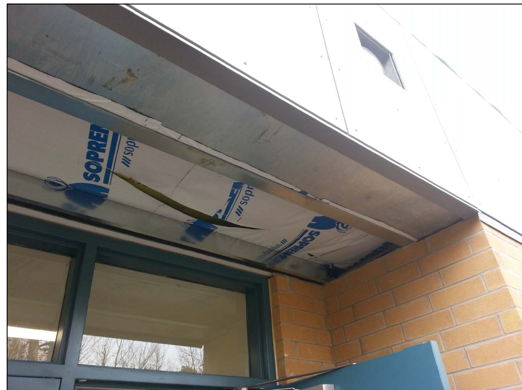
SOFFIT - DURING CONSTRUCTION FROM 2013
