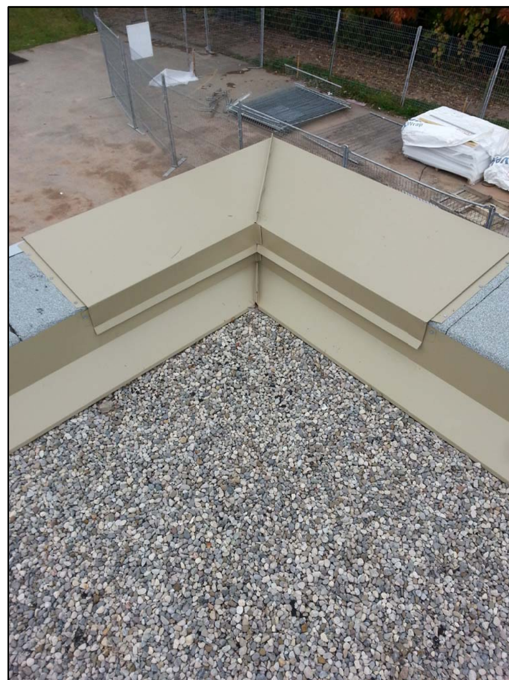
ROOF PARAPET - DURING CONSTRUCTION FROM 2013
