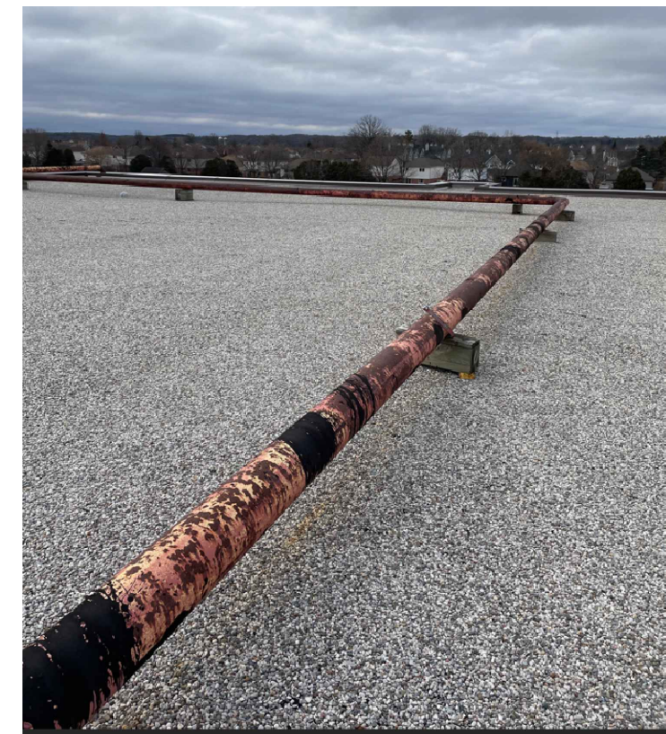
ROOF - GAS PIPING 5
