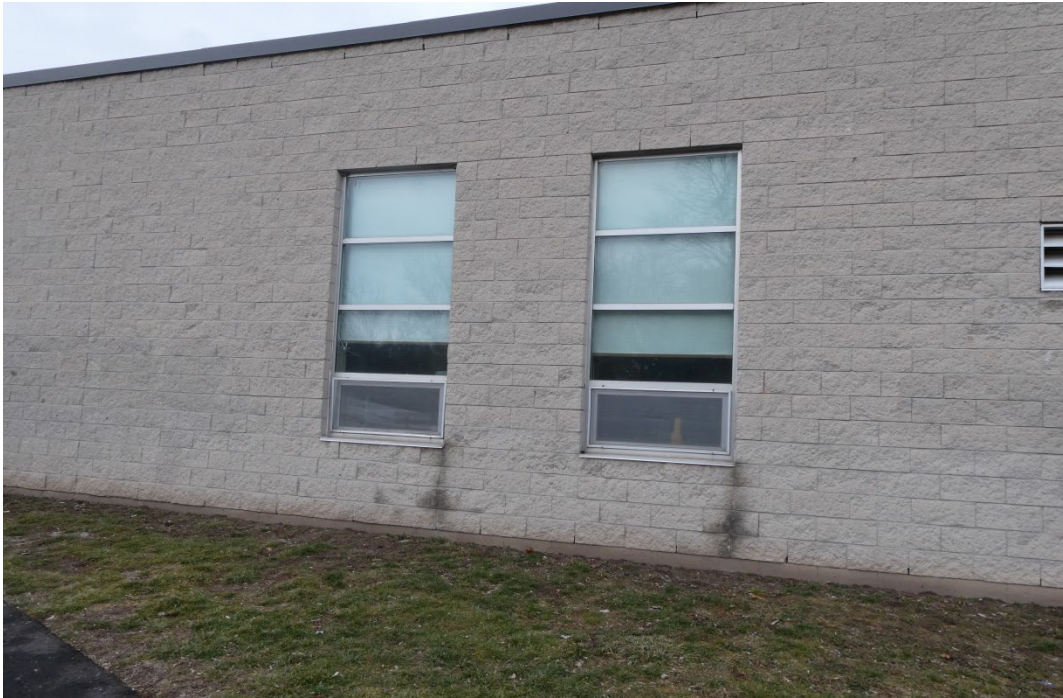
PHOTO #7 – VIEW OF WINDOWS PARTIAL SOUTH ELEVATION
