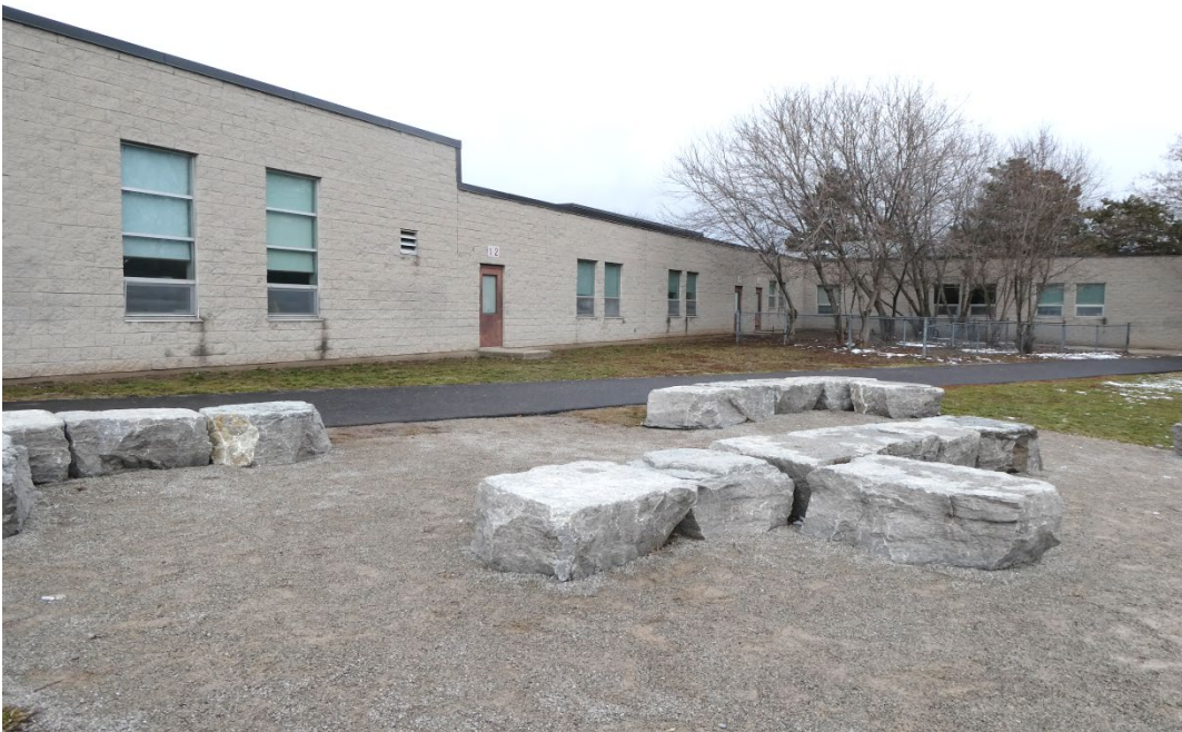
PHOTO #8 – VIEW OF WINDOWS SOUTH / WEST ELEVATION
