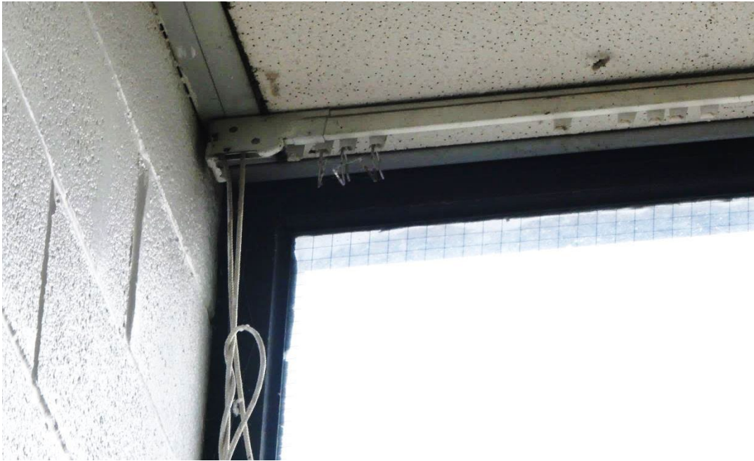
PHOTO #21 – TYPICAL VIEW OF HEAD & JAMB – WINDOW W2 THRU W6
