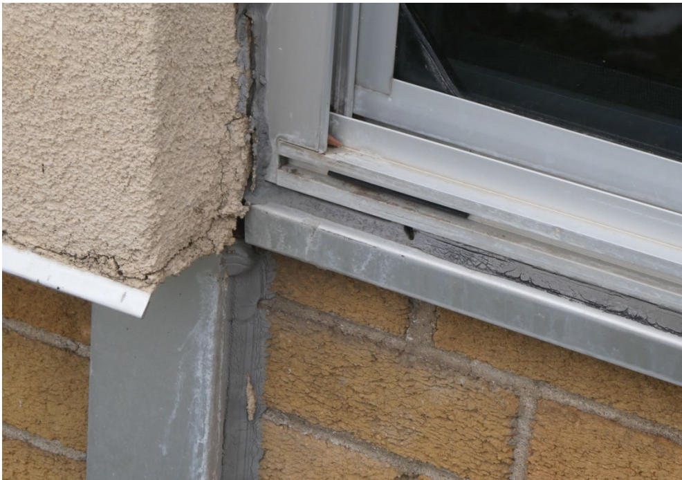
PHOTO #14 – VIEW OF EXTREME JAMB / SILL – WINDOW W1
