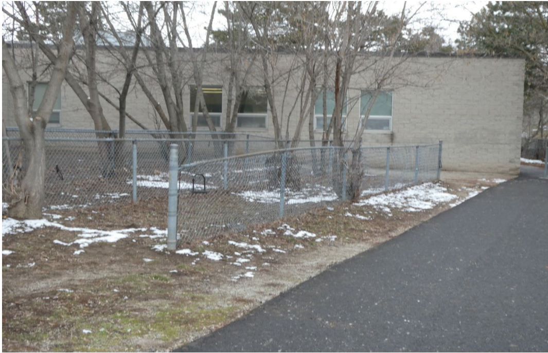
PHOTO #5 – VIEW OF WINDOWS PARTIAL WEST ELEVATION
