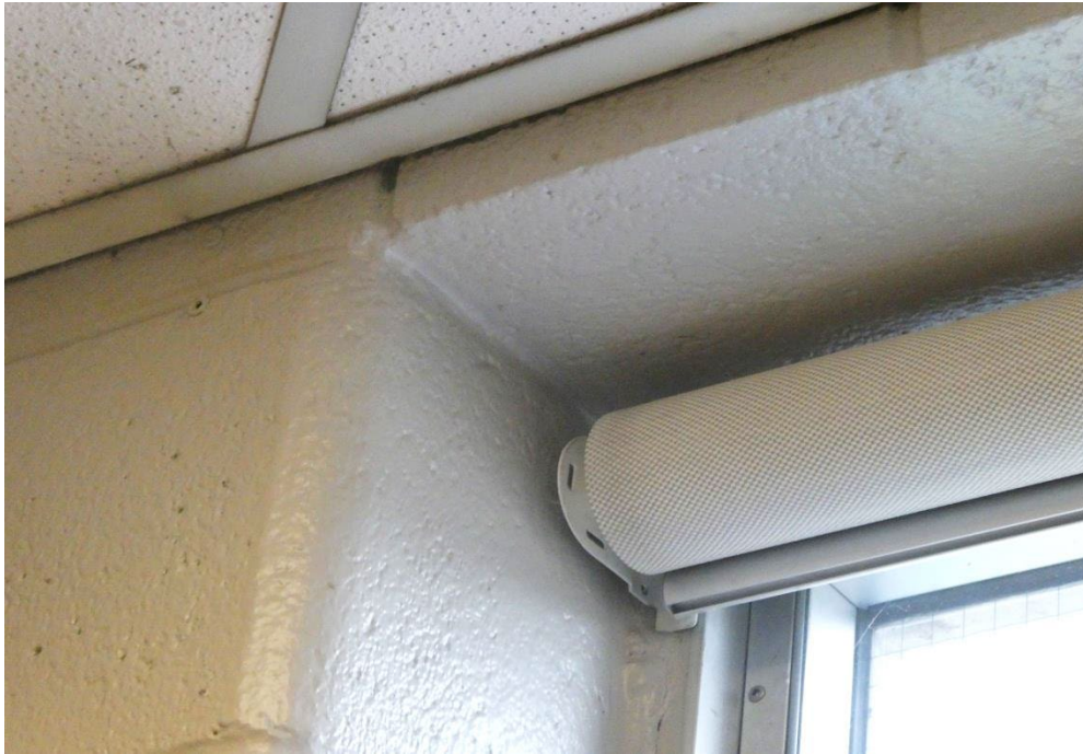
PHOTO #15 – INTERIOR VIEW OF HEAD / JAMB – WINDOW W1
