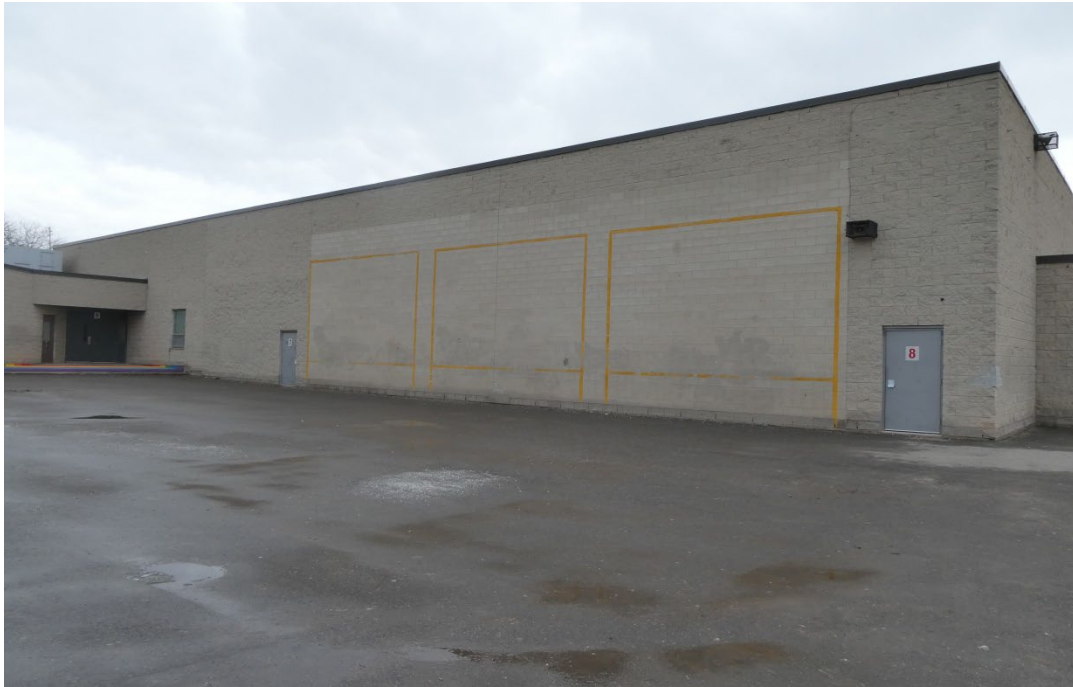
PHOTO #9 – VIEW OF PARTIAL NORTH (GYM) ELEVATION
