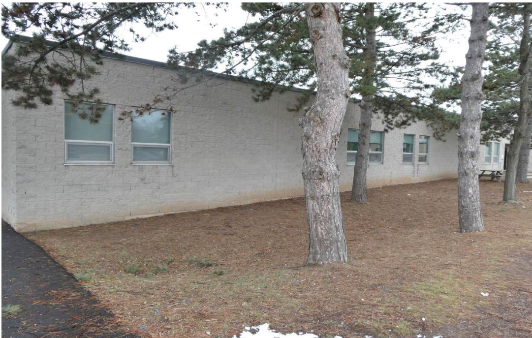
PHOTO #4 – VIEW OF PARTIAL EAST (FRONT) ELEVATION
