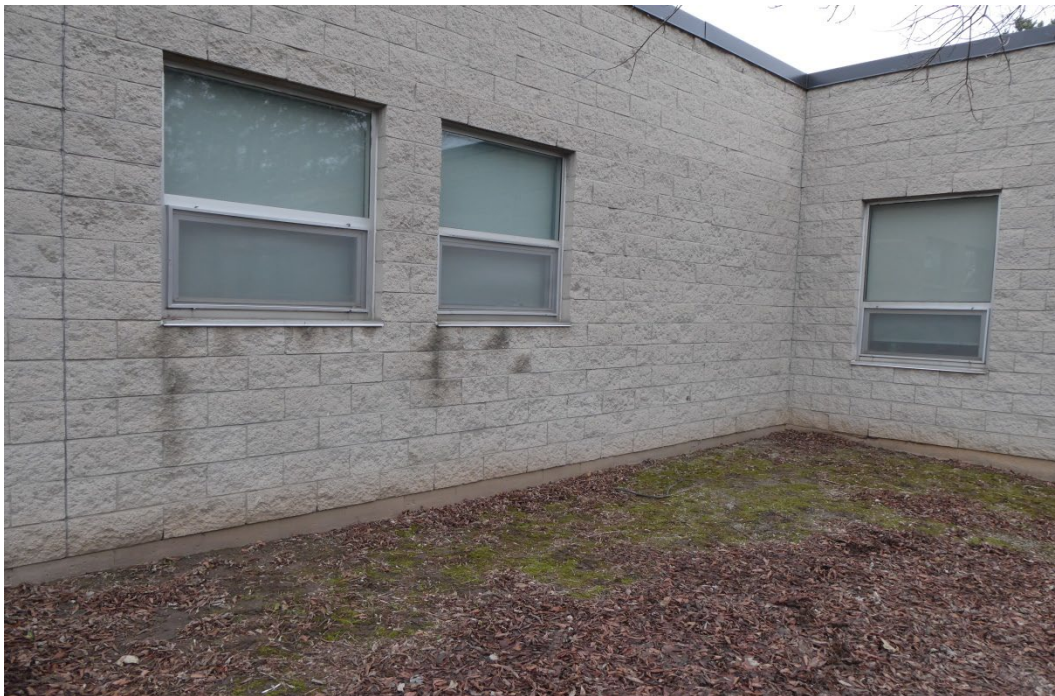
PHOTO #6 – VIEW OF WINDOWS PARTIAL SOUTH / WEST ELEVATION
