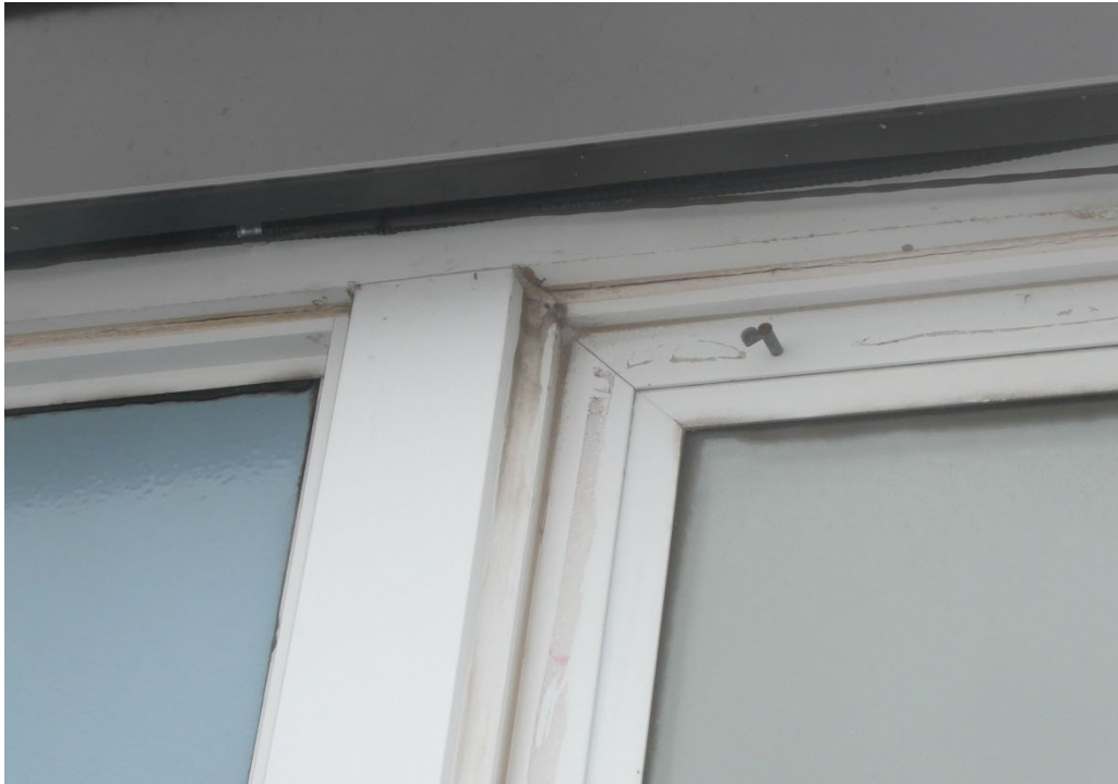
PHOTO #11 – TYPICAL VIEW OF HEAD @ MULLION - WINDOW W1
