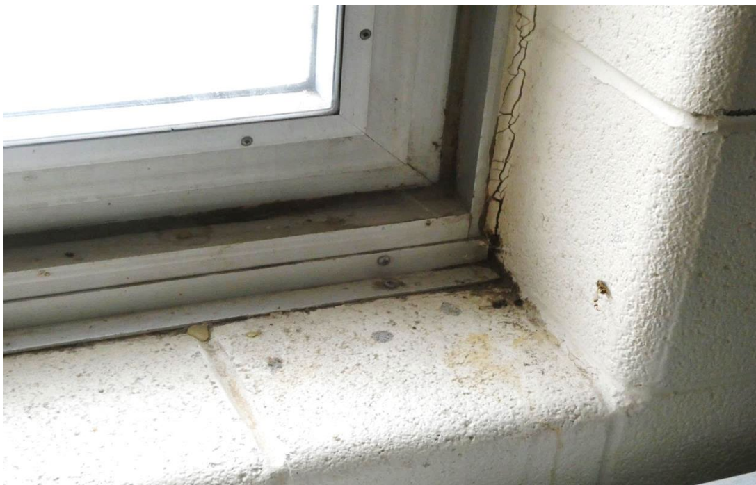
PHOTO #22 – TYPICAL VIEW OF JAMB / SILL – WINDOW W2 THRU W6
