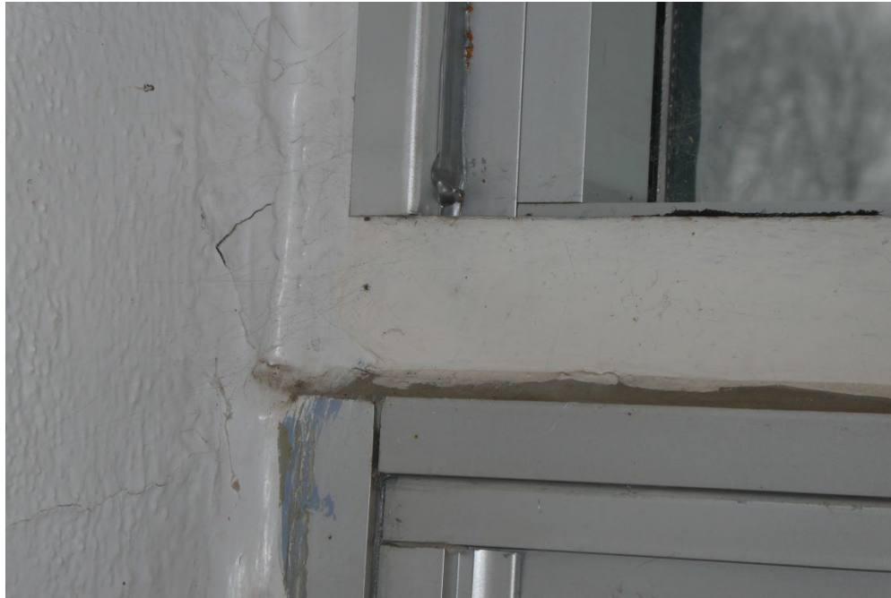
PHOTO #17 – VIEW OF HSS INFRASTRUCTURE MEMBER – WINDOW W1
