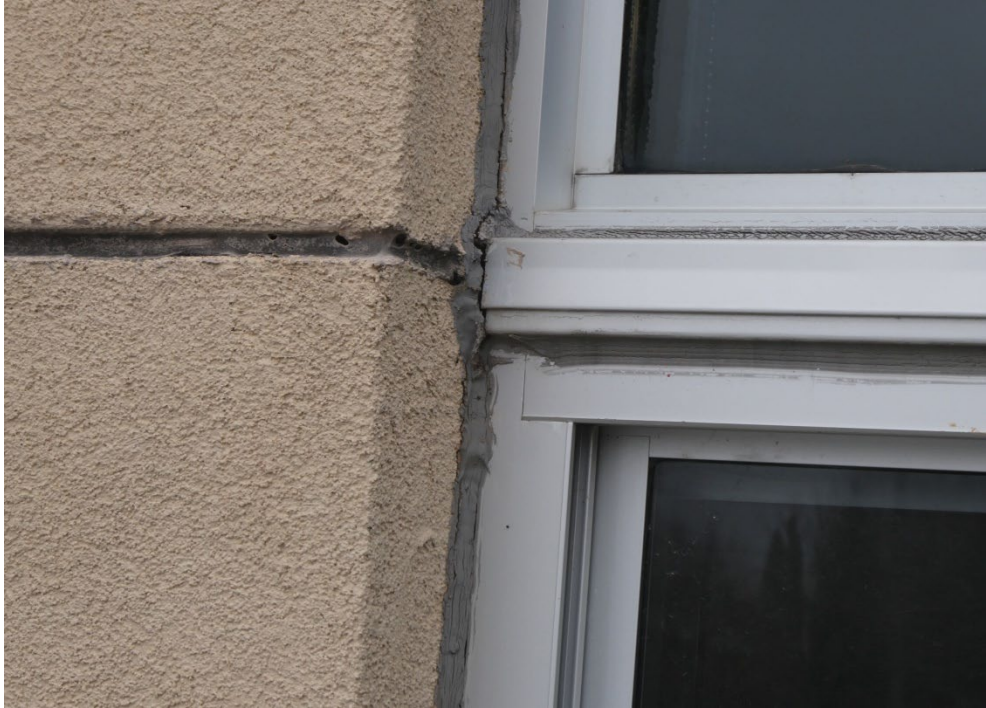
PHOTO #13 – EXTREME JAMBS @ MID MULLION – WINDOW W1
