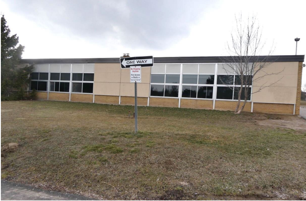
PHOTO #1 – VIEW OF WINDOWS PARTIAL SOUTH (FRONT) ELEVATION
