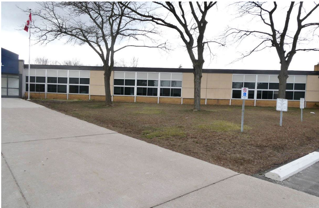
PHOTO #2 – VIEW OF PARTIAL SOUTH (FRONT) ELEVATION
