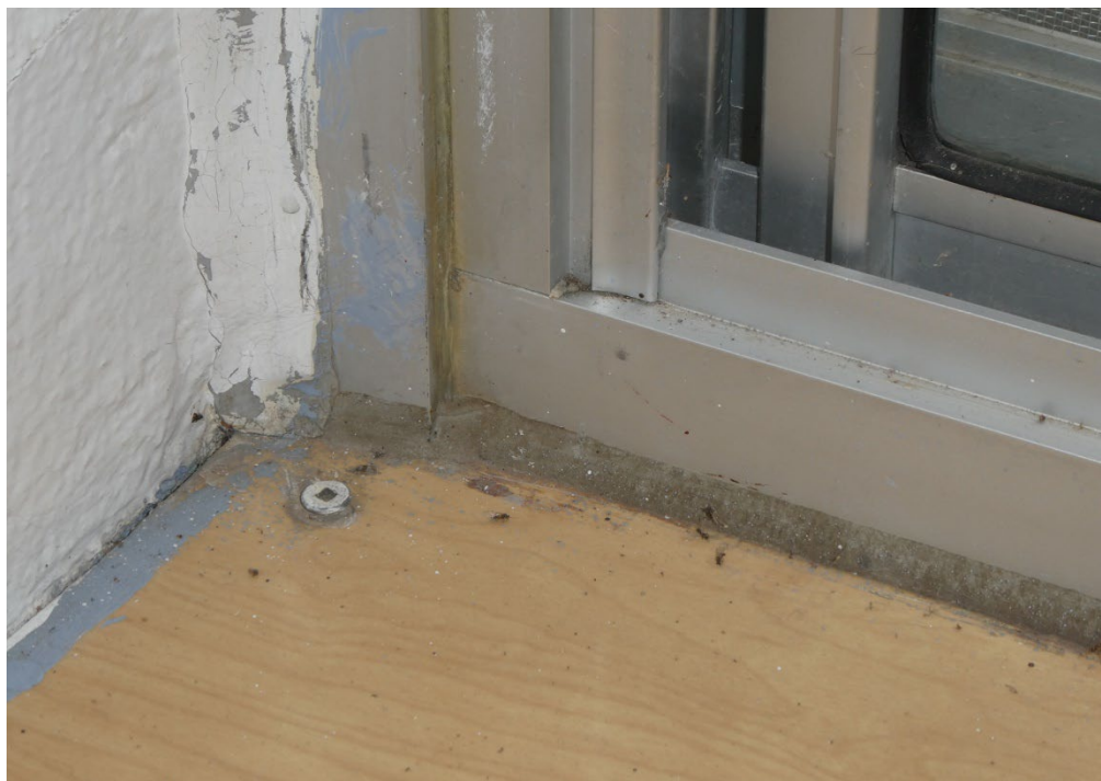
PHOTO #16 – INTERIOR VIEW OF JAMB / SILL – WINDOW W1
