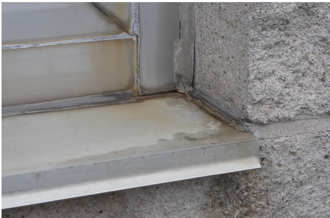
PHOTO #20 – TYPICAL VIEW OF JAMB / SILL – WINDOW W2 THRU W6
