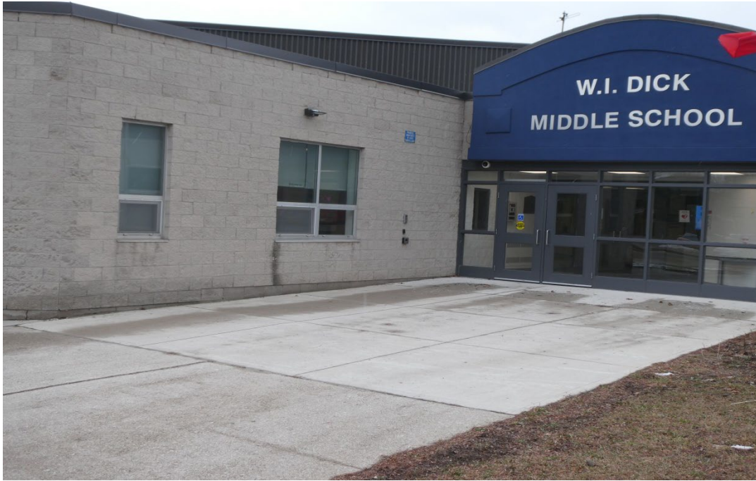
PHOTO #3 – VIEW OF WINDOWS NORTH ELEVATION (ADMIN. OFFICE)
