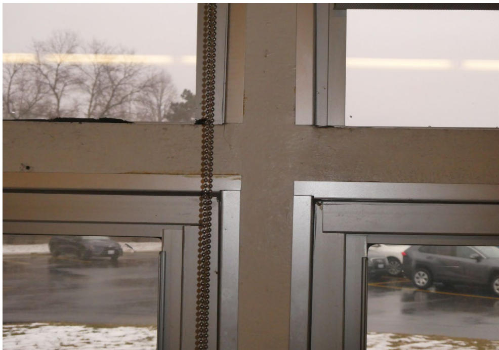
PHOTO #18 – VIEW OF HSS INFRASTRUCTURE MEMBER – WINDOW W1
