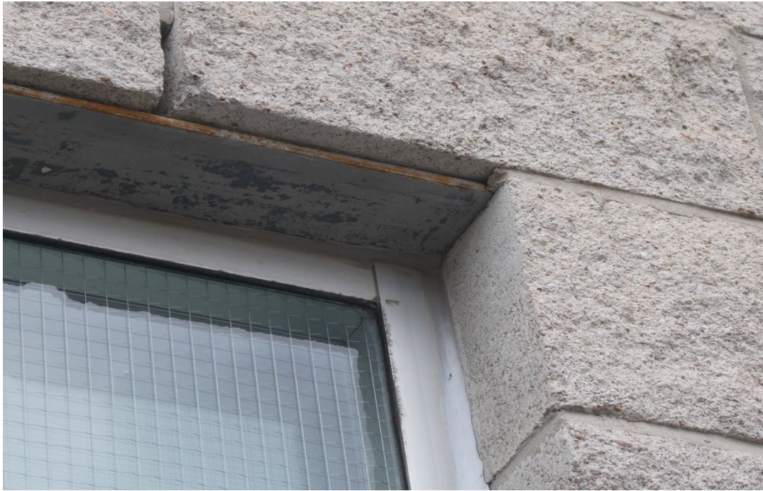
PHOTO #19 – TYPICAL VIEW OF HEAD & JAMB – WINDOW W2 THRU W6
