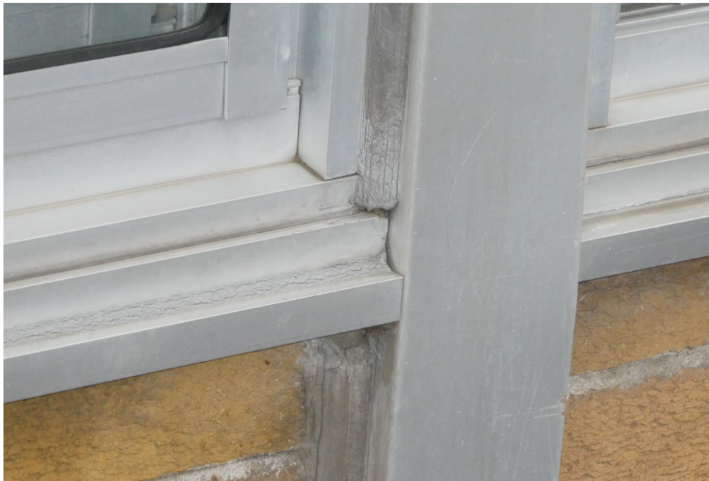
PHOTO #12 – TYPICAL VIEW OF SILL @ MULLION – WINDOW W1
