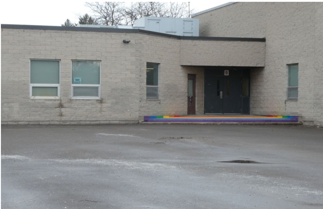
PHOTO #10 – VIEW OF WINDOWS PARTIAL WEST ELEVATION
