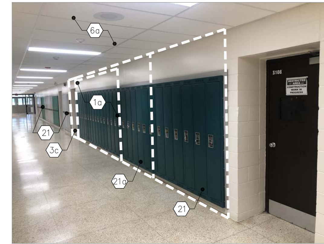
CORRIDOR OUTSIDE RM S108 & S107 SHOP - LOOKING TOWARDS SOUTH WEST
