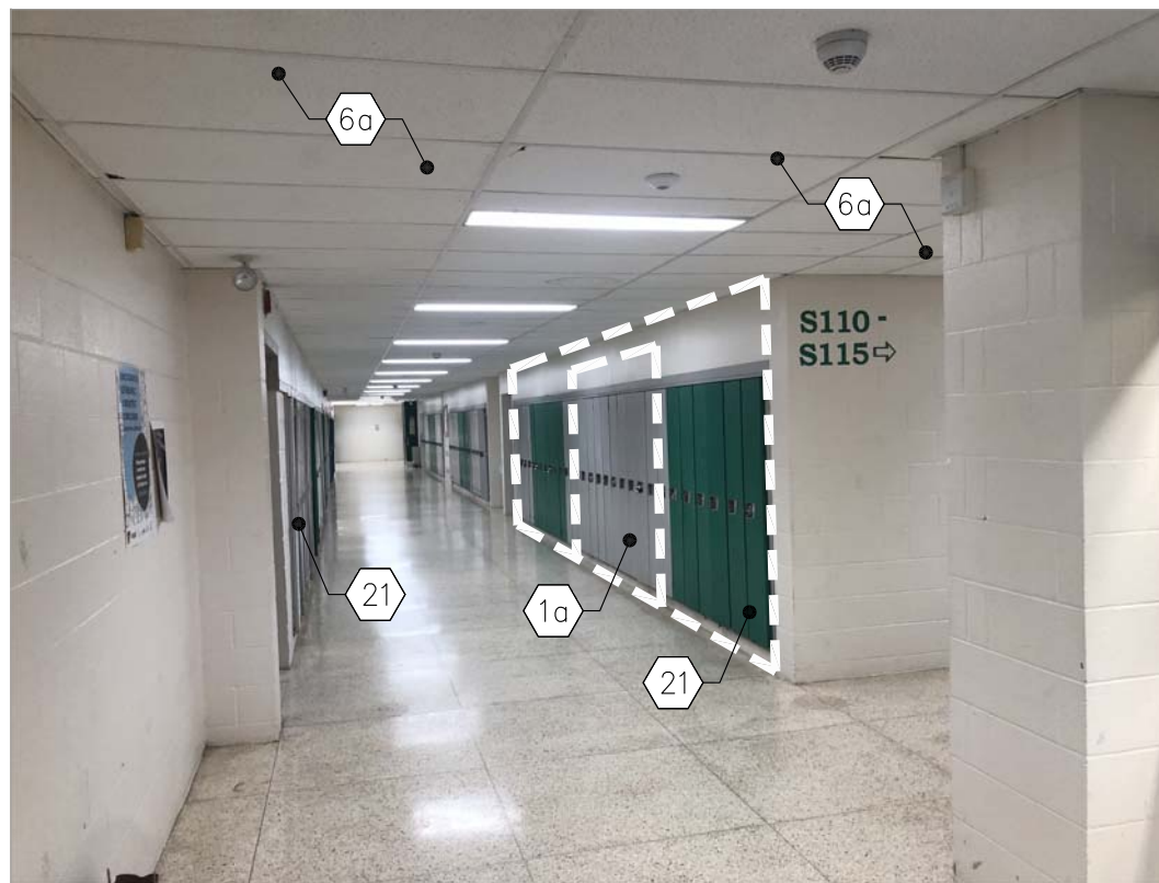
CORRIDOR OUTSIDE RM S110 SHOP - LOOKING TOWARDS NORTH
