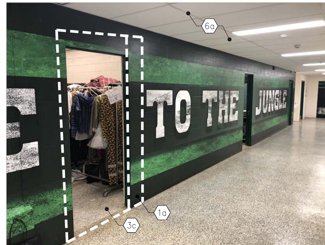
CORRIDOR OUTSIDE RM W111 - PARTIAL SOUTH WALL
