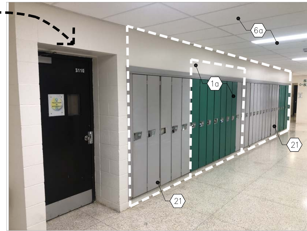
CORRIDOR OUTSIDE RM S110 SHOP - LOOKING TOWARDS SOUTH EAST
