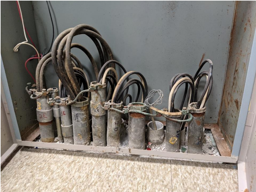
LABELLED PULL BOX IN ROOM 6-22
