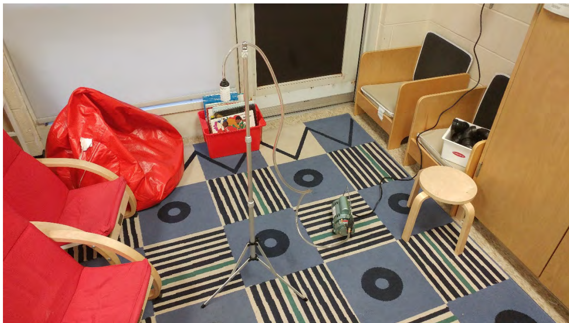
Photo 1: Air monitoring equipment, Room 17
